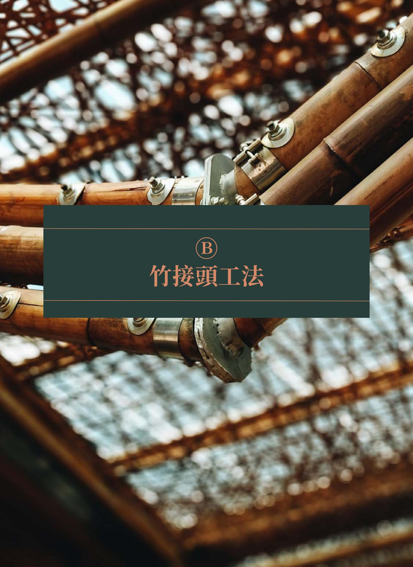
A close-up photograph of several bamboo poles joined together using metal fittings. The fittings consist of cylindrical sleeves with flanges and bolts. The bamboo has a natural brown color and a visible grain. The background is a blurred lattice structure, likely part of a traditional building's roof or ceiling.
